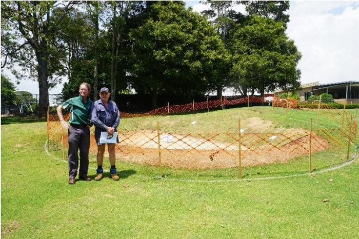
Wayne and Jimmy are discussing the finer points of bunker construction. The new design provides more of a feature and will lessen the amount of sand that is blown out of the bunker by the strong westerly winds that blow in early spring.
